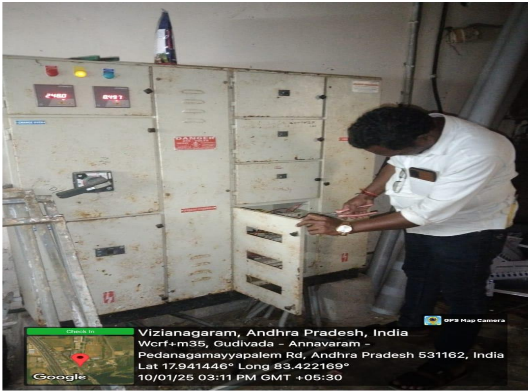
Solar Panel Board Repair
