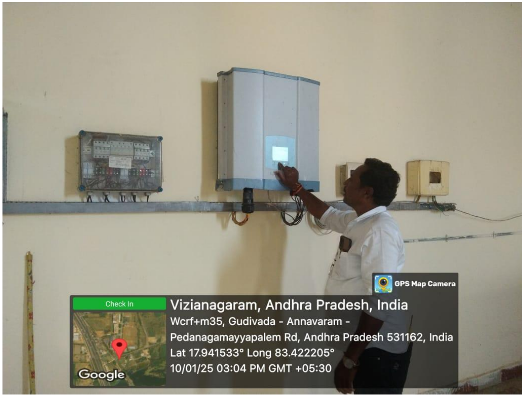
Solar Panel inverter repair
